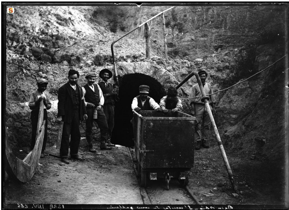
Galleria e vagone (Sardinia Digital Library).
